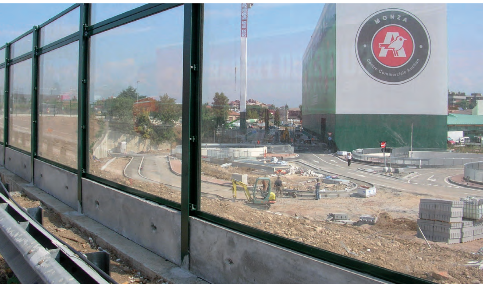
Barriera antirumore costituita da pannelli in cemento precompresso alla base e polimetilmetacrilato in elevazione. Noise protection safety barrier made of pre-stressed concrete and polymethylmethacrylate (PMMA).
