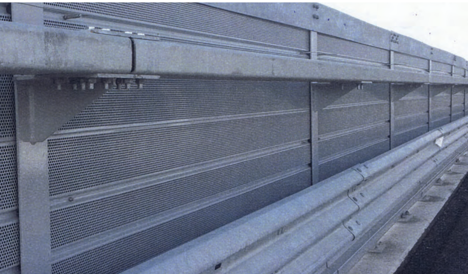
Barriera bordo ponte classe H4 integrata con pannelli antirumore. H4 class side bridge safety barrier with noise protection panels.
